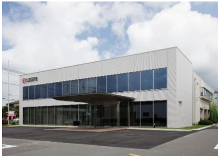
Exterior view of Kyocera's Kagoshima Sendai plant
